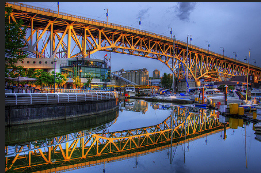
Granville Street Bridge, Vancouver, seismic retrofit : 1996
